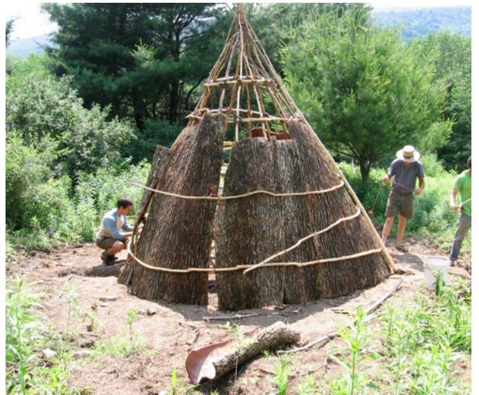
Left: Assembling the Camp Lean To, from cut northern white cedar logs. Below: Large sheets of elm bark goes on the Wickiup.
